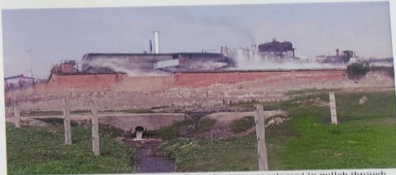
Plate 13: The effluents from Roza Sugar Factory are released in nullah through pipes.
