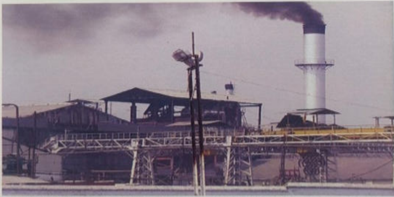
Plate 12: The untreated effluents discharged from the factory cause pollution in Khannaut river
